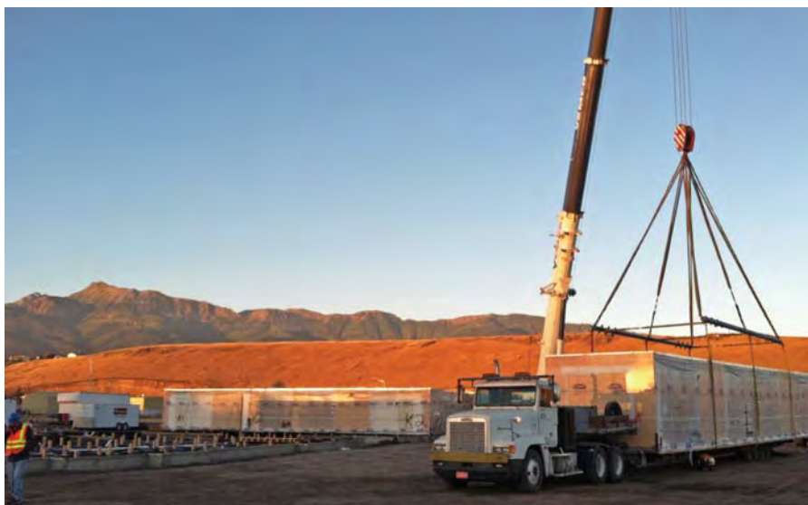
Oversize load getting ready for transport by Modern Building Systems. These types of loads will now have more direct access to I-5 because of the improved vertical clearance.
